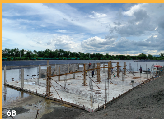
Figure 6A. Pond reconstruction showing pond bottom leveling 6B. Slab construction with rebar posts 6C. Construction nearing completion
