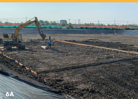
Figure 6A. Pond reconstruction showing pond bottom leveling 6B. Slab construction with rebar posts 6C. Construction nearing completion
