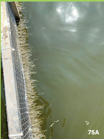
Figure 75A & B. Floating fecal strands attach to confinement gates, but they can be collected by diverting them to the wall where they can be manually removed.
