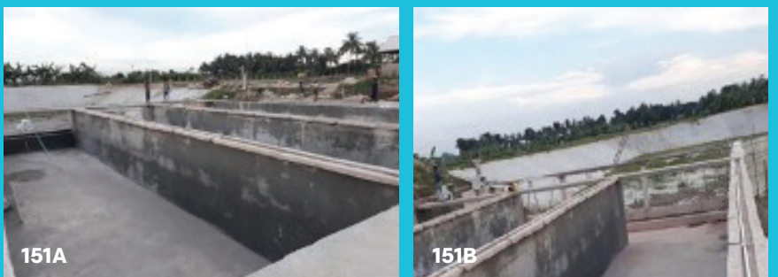
Figure 151A & B. Raceway cell and baffle wall
