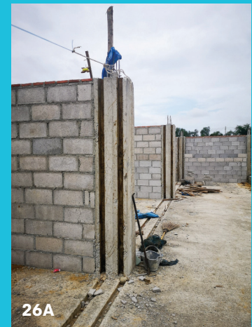
Figure 26A & B. Confinement gate slots
