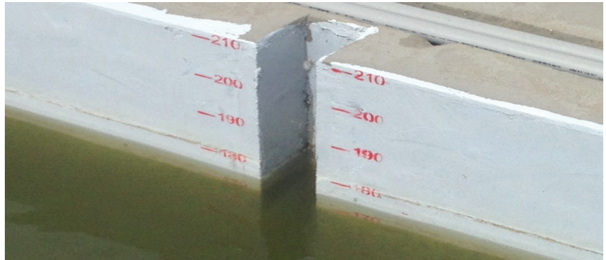
Figure 80. Careful calculation of the raceway volume using depth markings on the walls and accurate amount of chemical treatments are critical.
