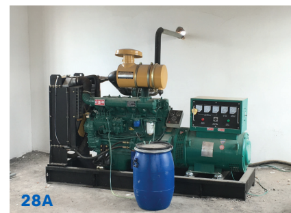
Figure 28A & B. Auto-start back-up electricity generators
