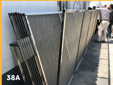
Figures 38A & B. Confinement gates prepared and installed in Vietnam
