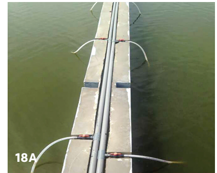
Figure 18A & B. Slots for supplementary air delivery system
