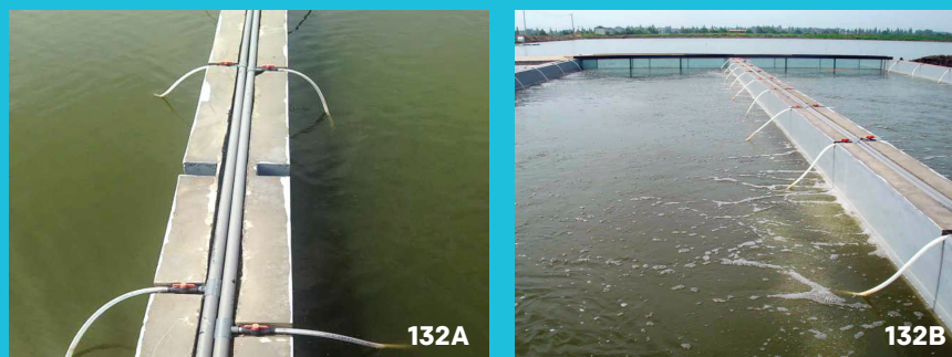
Figure 132A & B. Supplementary aeration device at IPRS raceway bottom
