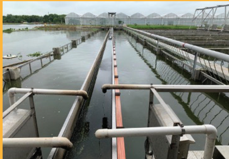
Figure 127. IPRS automatic double suction device (6 m QZ, new design)
