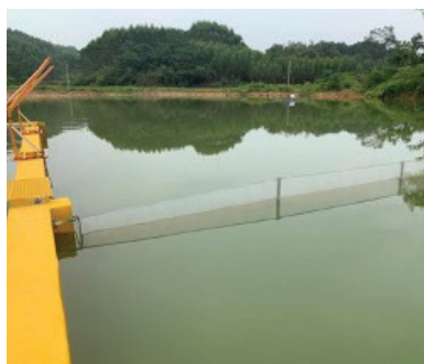
Figure 135. Baffles for IPRS operation
