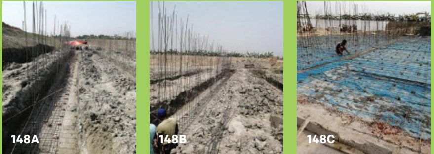
Figure 148A – C. Foundation & flooring work in progress
