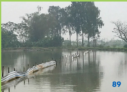
Figure 89. Poorly installed baffle, not likely to function correctly Figure 90A & B. Well-built and properly installed HDPE baffle
