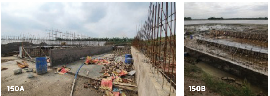
Figure 150A & B. Raceway cells under construction
