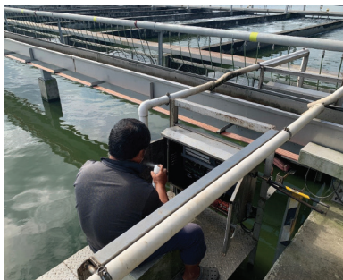
Figure 86. Maintenance of IPRS programmable waste removal gears
